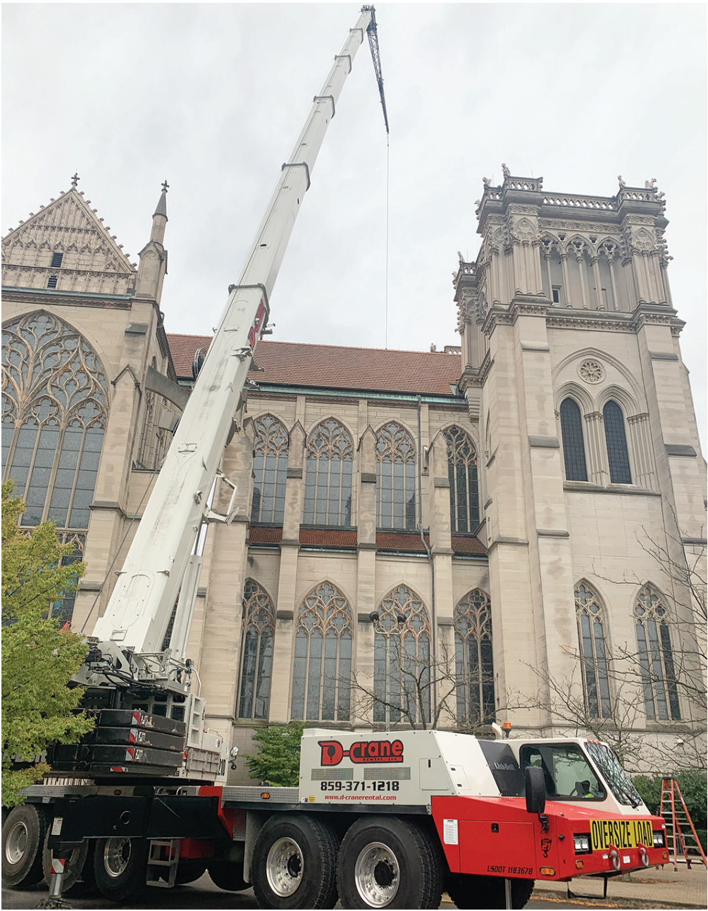
(above) A bucket attached to 250-foot crane suspends architects from SHP as they painstakingly scan every inch of the Cathedral Basilica of the Assumption mapping out every crack and crevice in need of repair. (top, right) A photo of a chimera atop the Cathedral illustrates the need for complete replacement. (center, right) Toward the middle of the Cathedral’s façade are a series of balustrades and colonnades whose metal pins have rusted requiring complete restoration and replacement. (bottom, right) Facing stones and carved details of the Cathedral are constructed from Indiana limestone. Many have cracked or shatter due to water damage.
