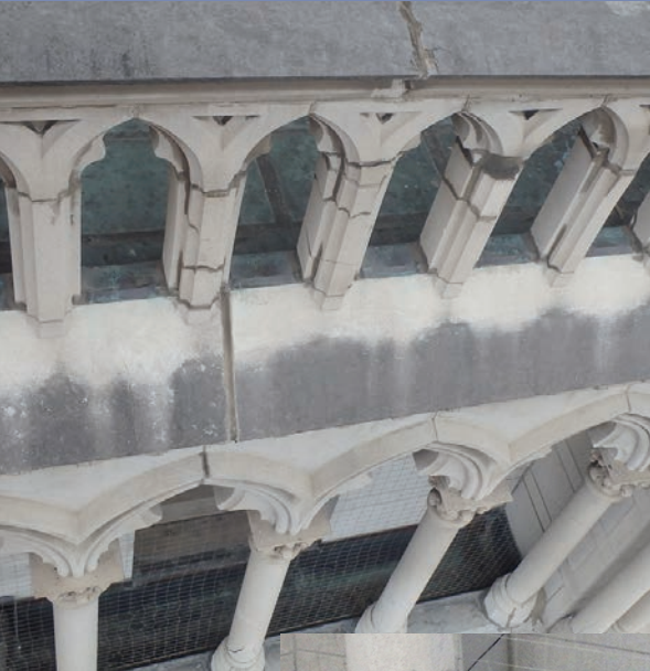
(above and right) Metal pins holding these stone arches and columns together have rusted from water damage, requiring their complete restoration by replication and replacement.
