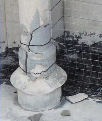
(above and right) Metal pins holding these stone arches and columns together have rusted from water damage, requiring their complete restoration by replication and replacement.
