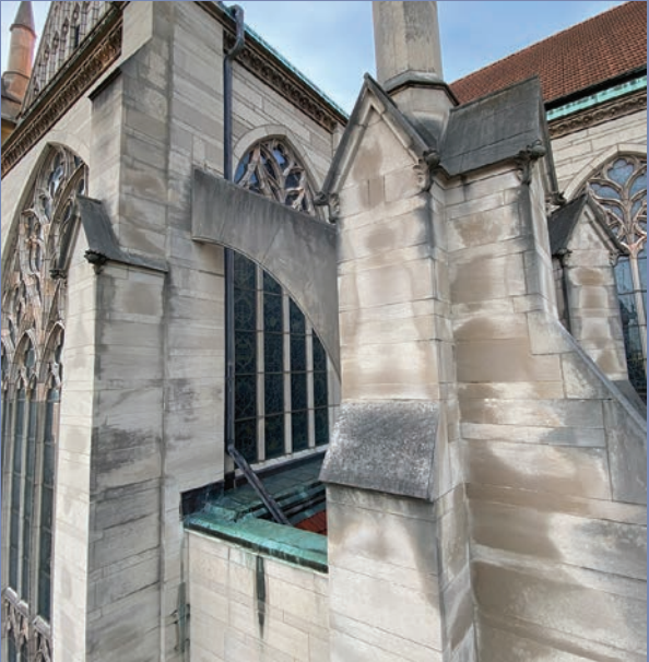
(above) Visible at numerous places across the exterior are dark stains from biological and carbon soiling. If left uncleaned and untreated, these areas will lead to future deterioration.
