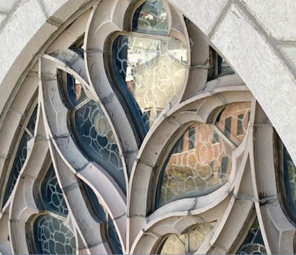
(below) Several windows are in need of conservation along with masonry repairs at the tracery frames that support many of the stained-glass panels.
