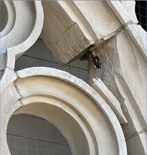
(below) Many of the solid Indiana limestone facing stones, and carved details of the Cathedral have cracked or shattered due to water damage, requiring complete replacement. In addition, extensive tuck-pointing, cementitious grout, and pin repair to jointed stones is required.
