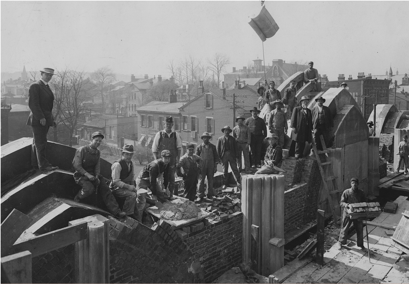
Construction of the stone façade began in 1908 and was completed in 1910. This photograph from 1909 to the left captures a view toward the west as workmen hoist stone for the façade into place. Such intricate movements required the work of many hands, from engineers and masons to skilled laborers and craftsmen.
