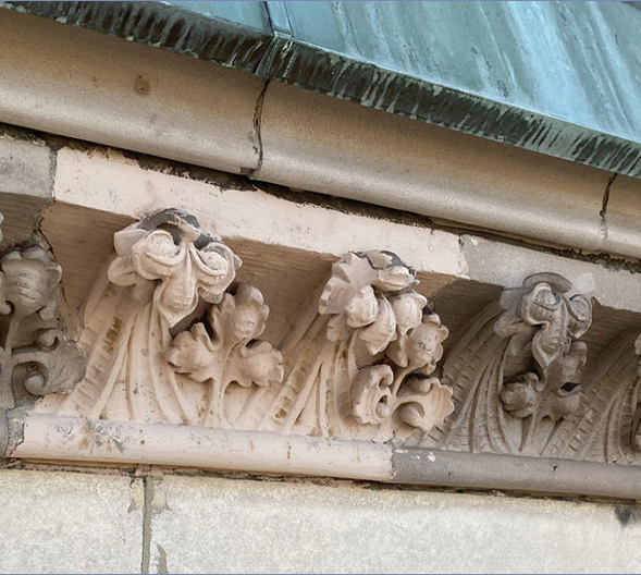
(above) The Cathedral features delicate carvings such as friezes and moldings. In many instances, water has permeated their seams, requiring restoration or complete replacement.
