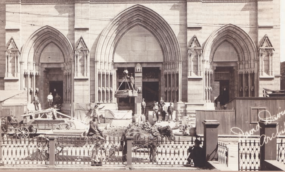
By Winter 1908, work on the lower facade was complete and attention shifted to the remaining upper half. In this photograph from early 1909, workmen pose as newly carved stone arches are prepared to be hoisted into place.
