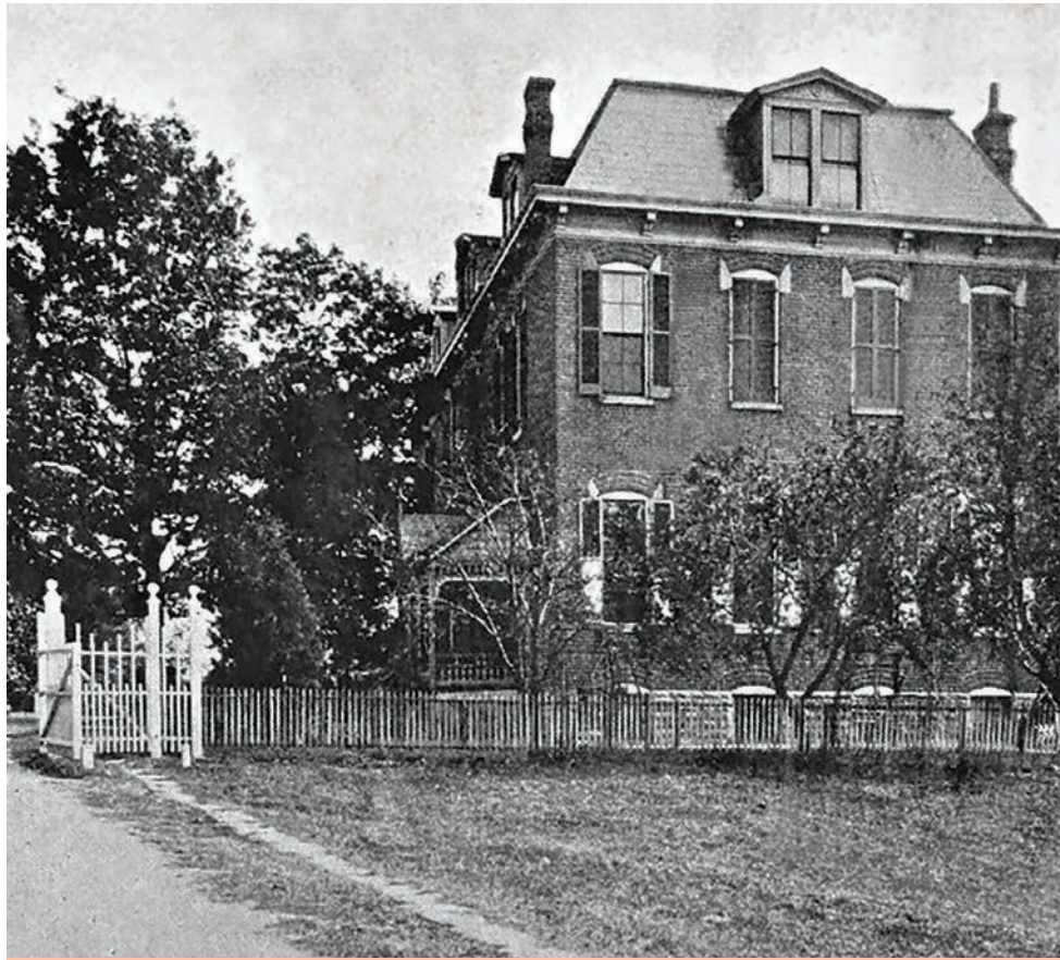
(above) The south annex built by Bishop Maes in 1892 to house the boy’s dormitory and living quarters for the resident chaplain, house physician, and Benedictine Sisters. (Courtesy of DCCH)
