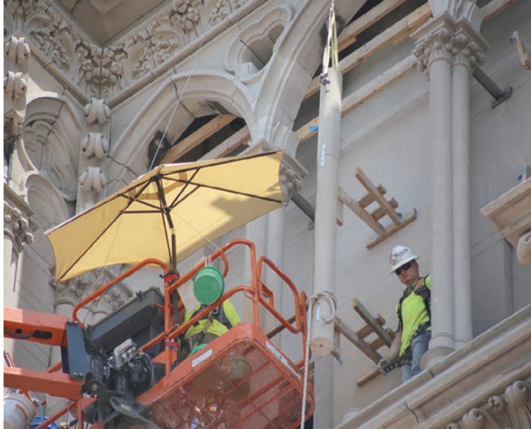
These two photos show a column being lifted to its home on the Cathedral’s façade. At left, Rob Davis, foreman, mans a rope keeping the column from crashing into the Cathedral as colleagues in a boom lift receive it. In an interview Mr. Davis quipped, “I felt like I was the horse sometimes.”
