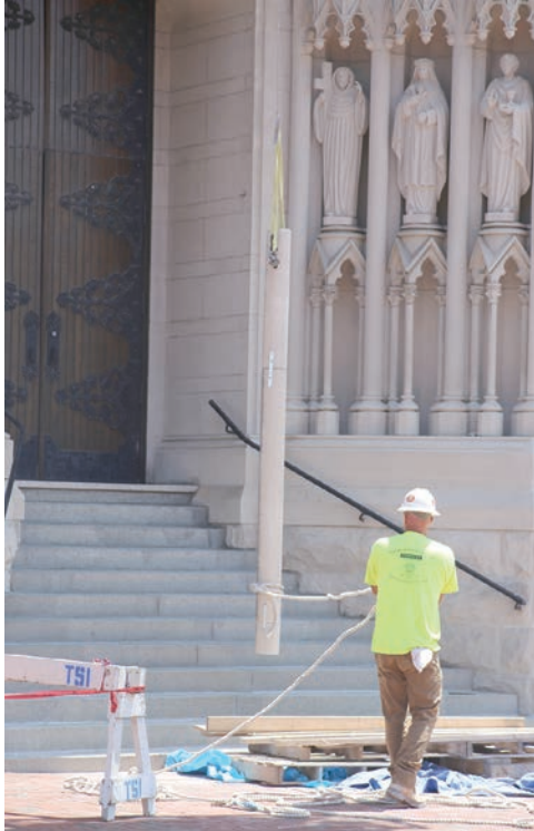
These two photos show a column being lifted to its home on the Cathedral’s façade. At left, Rob Davis, foreman, mans a rope keeping the column from crashing into the Cathedral as colleagues in a boom lift receive it. In an interview Mr. Davis quipped, “I felt like I was the horse sometimes.”
