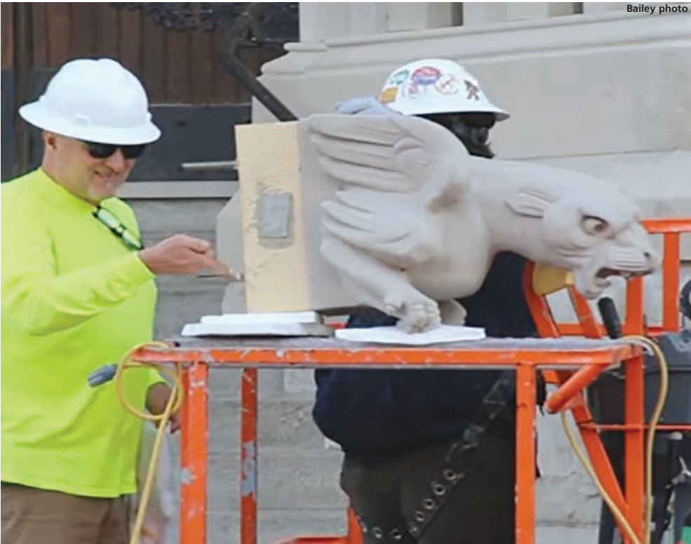
Rob Davis of Trisco Systems prepares the final gargoyle for hoisting.
